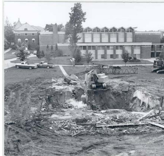
Figure 5: Bulldozing the site in 1972
